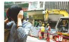
Construction of Building
